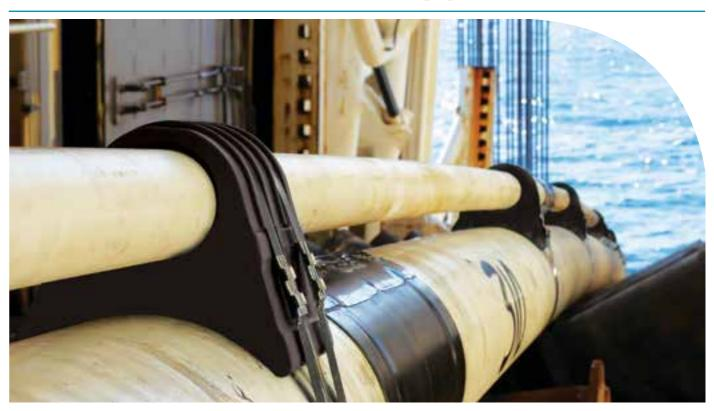
KOHRANG Piggyback Saddles are applicable in the oil and gas industries. This product correctly places smaller pipelines on the main lines. In other words, the aim is to facilitate the installation of the pipe system at the either offshore or onshore areas. KOHRANG Piggyback saddle advantages:
