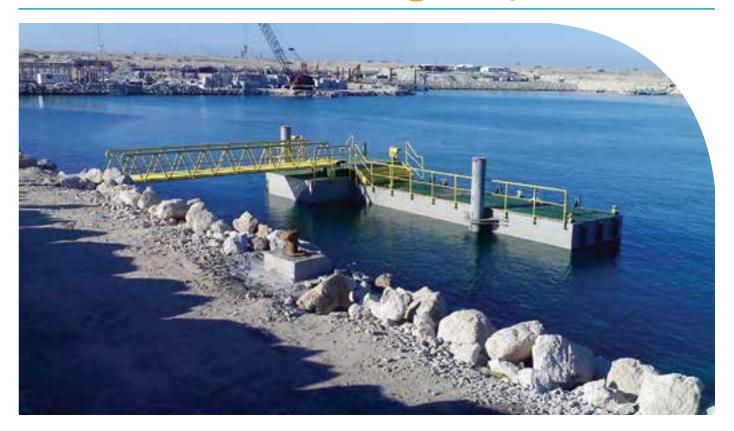
A type of marine structure used at the locations with low water depth. They install alongside the passenger, cargo, and fishing quays, where various types of vessels berth at a pontoon to unload their passengers or cargos. Then, the unloaded passengers or cargos could be transferred by a ramp or other access ways to the in-land area. Floating jetties are applicable for sailing ports, and passenger, recreational, and fishing quays.
